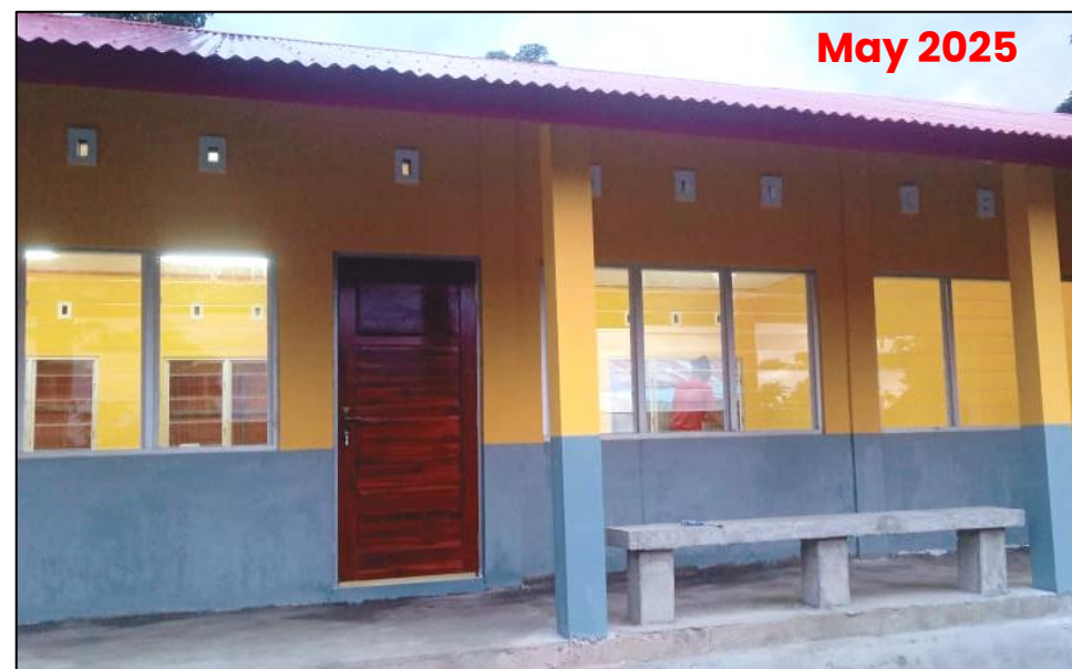
"Moris Foun 2" Pre-School rebuilt in 4 months (2025)
