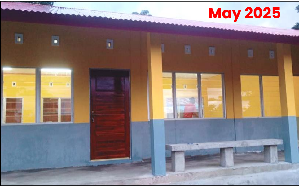
"Moris Foun 2" Pre-School rebuilt in 4 months (2025)
